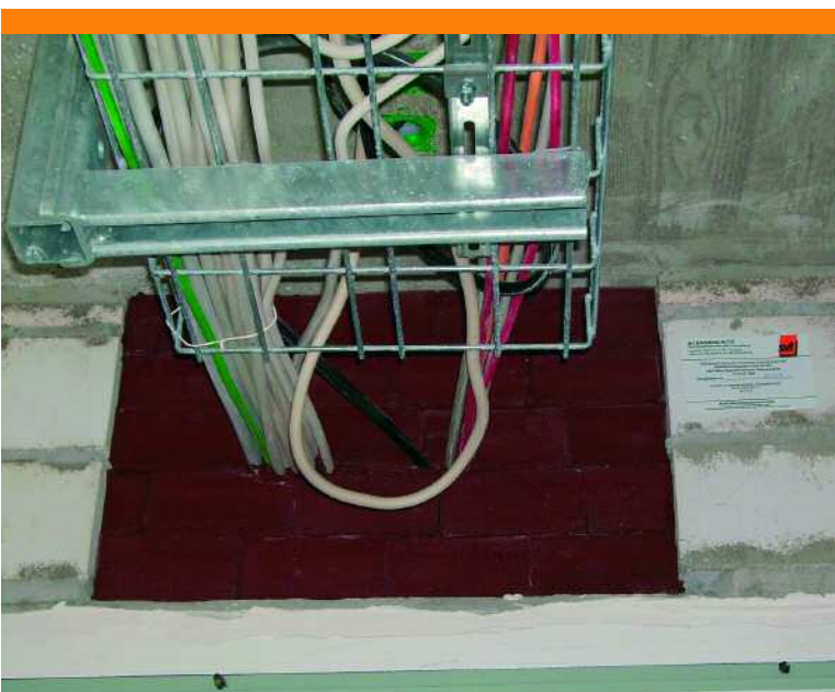
PYRO-SAFE Steinschott COMBI 170 S90 PYRO-SAFE Block Bulkhead COMBI 170 S90
