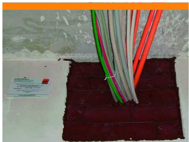
PYRO-SAFE Steinschott 120 S90 PYRO-SAFE Block Bulkhead 120 S90
